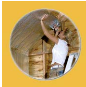
Fig. 6 – Radiant Barrier Systems
